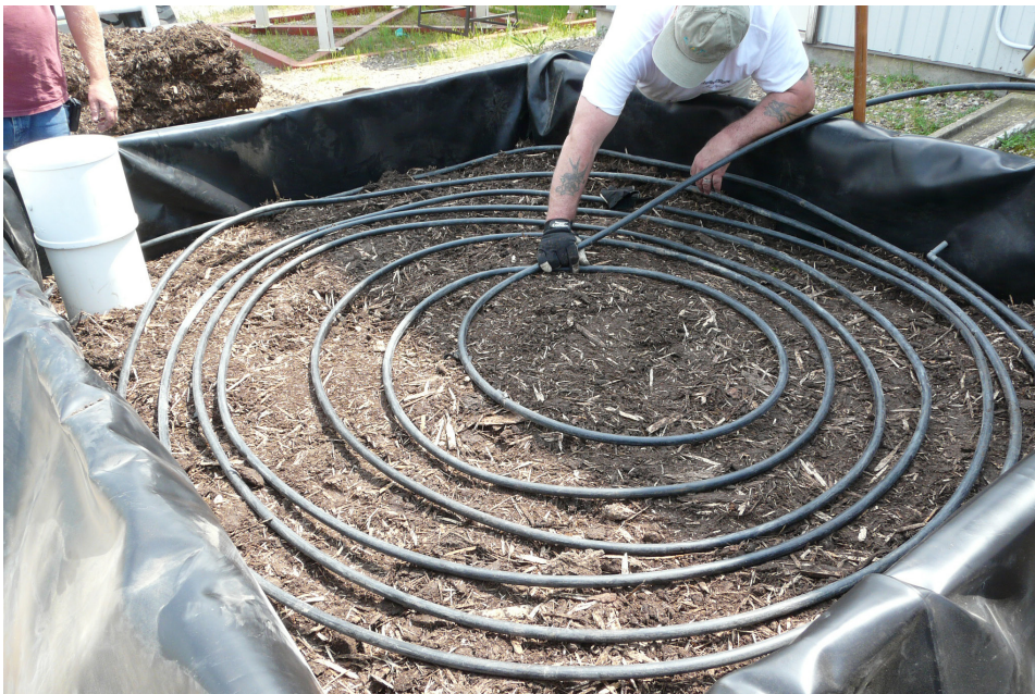
Figure 8. Install heating coil in the biomix layer 20 centimeters above the gravel
