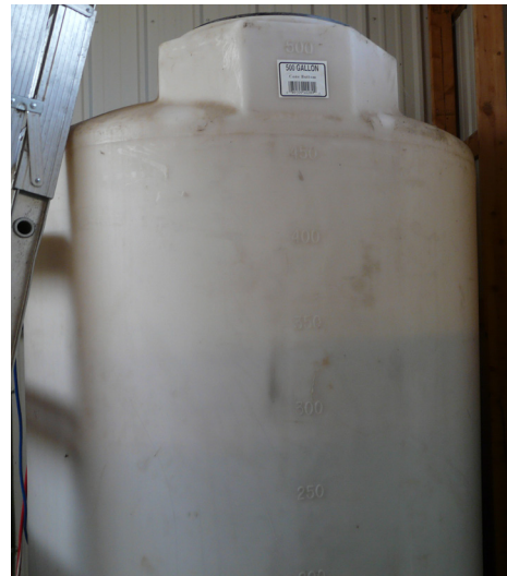
Figure 4. Pesticide rinsate storage tank
